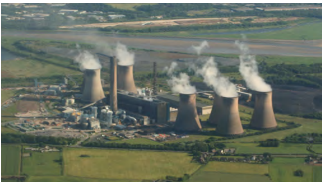
Figure 1 - SSE's "Fiddlers Ferry" coal fired power plant in Cheshire to be closed by the end of March 2020
