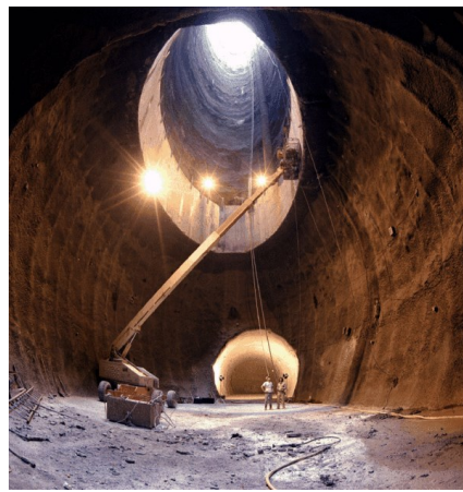
A part of the 87.1 km long tunnel under construction
